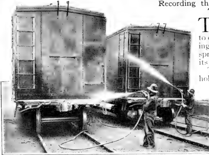
The paint is first vaporized and then forced through hose and sprayed on the cars by means of compressed air
